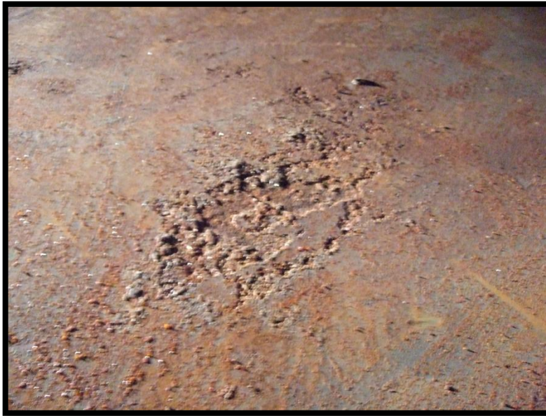
Floor plate corrosion
