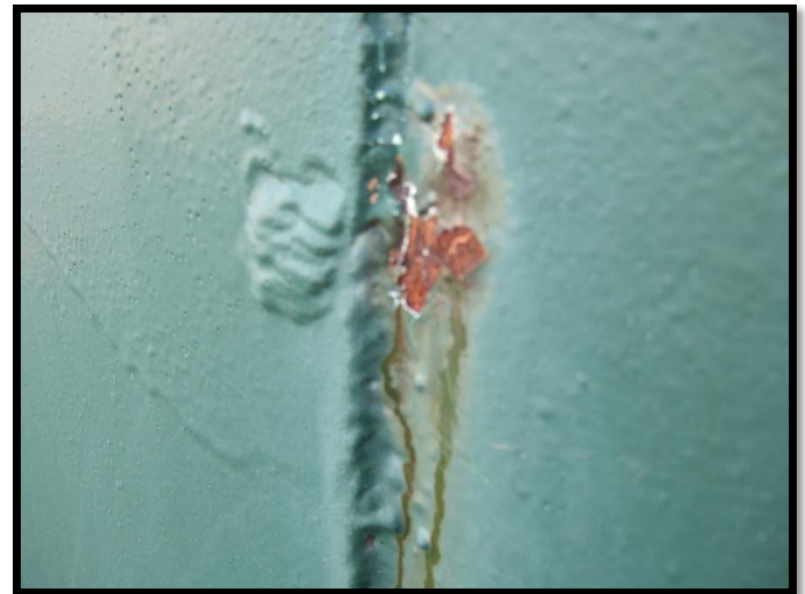
Lap-welded seam leak
