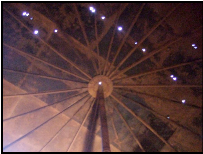
Severe roof corrosion
