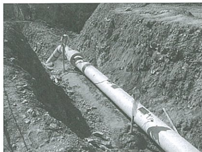
Electrodes used to monitor pipe potential
