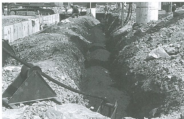
Laying of flexible anode
