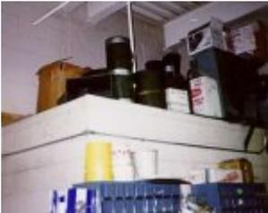
You are conducting a walkaround safety inspection when you notice the guardrail along an elevated platform area is missing. As you now understand, the missing guardrail represents a hazardous condition and would be considered a surface cause if an accident occurred. But it also represents a symptom of a deeper problem...a root cause...a system weakness: What might that be? Use the accident weed to figure that out.
