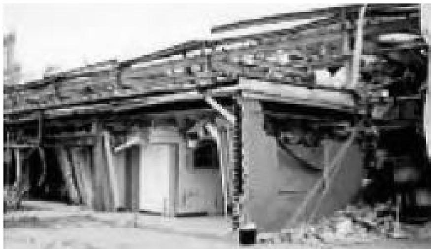
Figure 3.26. Damage to Flixborough control room.
