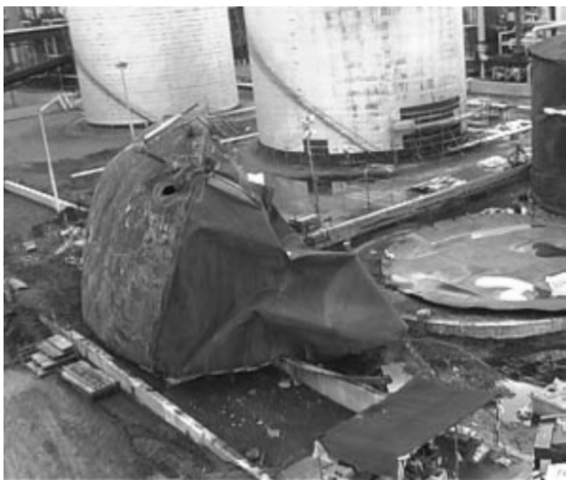
Figure 2.6. Collapsed tank at Motiva refinery, courtesy CSB.
