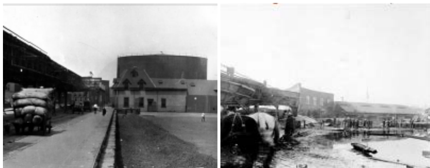
Figure 5.29. Molasses tank failure; before and after.
