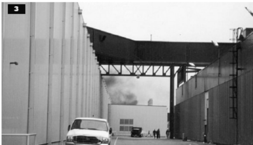
Figure 5.31. Cloud of nitric oxide and nitrogen dioxide.
