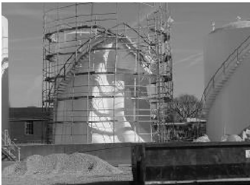
Figure 5.32. Tank collapsed by vacuum.
