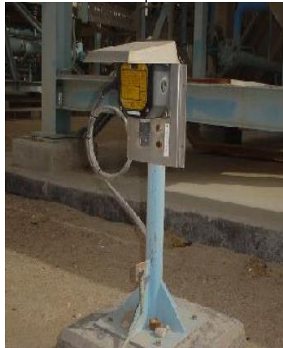
FIXED SENSORS DETECTS 10 PPM OF H2S
