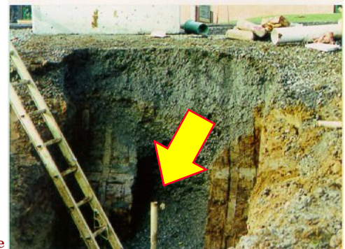
Watch for impalement hazards at base
