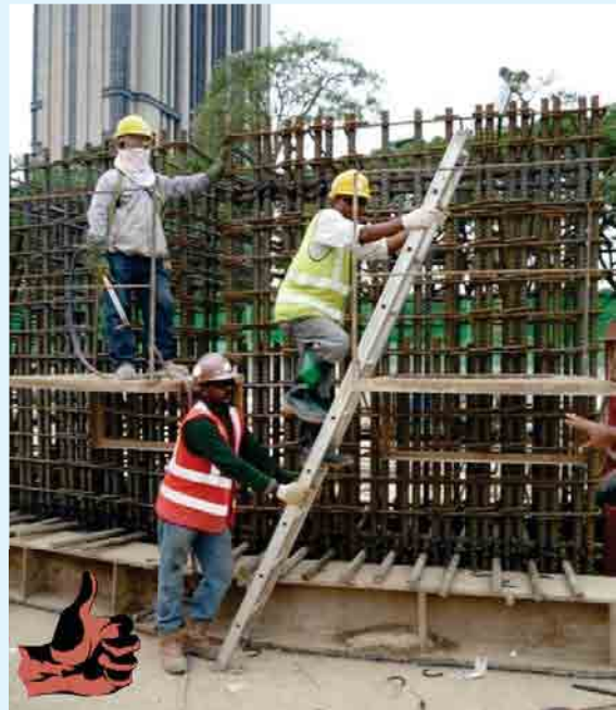
Ladders should be secured during use
