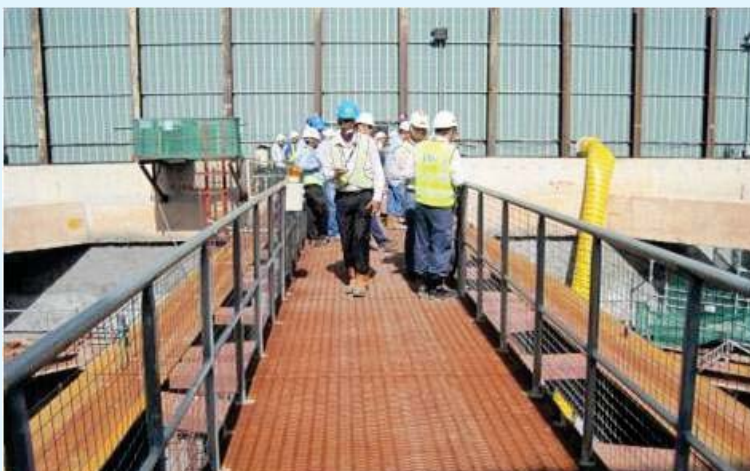
Provision of secure foothold and handhold
